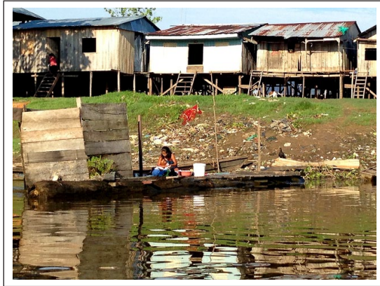
Figure 16. Photo of the main frontal view of the newly formed neighborhood Fantasy Island housing, Leticia, Colombia. Houses are developed onto pilotis clad with wood planks and galvanized steel/zinc plates on walls and roofs. © Maria Paz Gutierrez.
