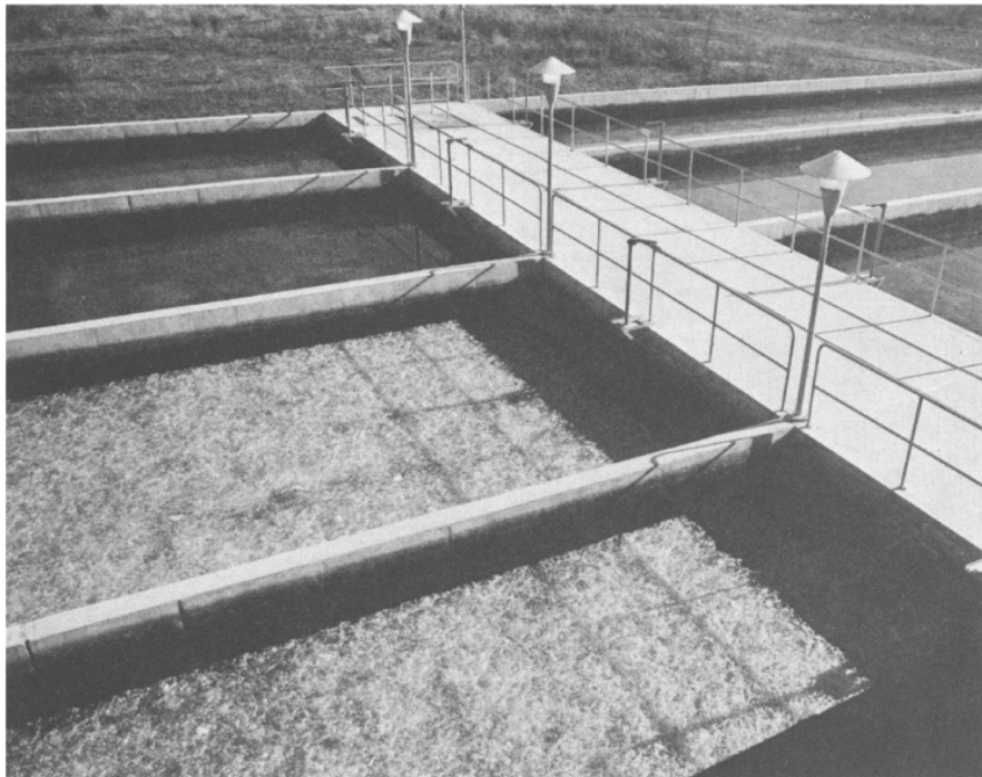
FIGURE 6—There are eight filter beds at Mad River Hatchery. Bubbles can be seen on the surface of the two ponds in the foreground as air surges up through the filter as part of the cleaning process. Photograph by George Bruley, 1973.
