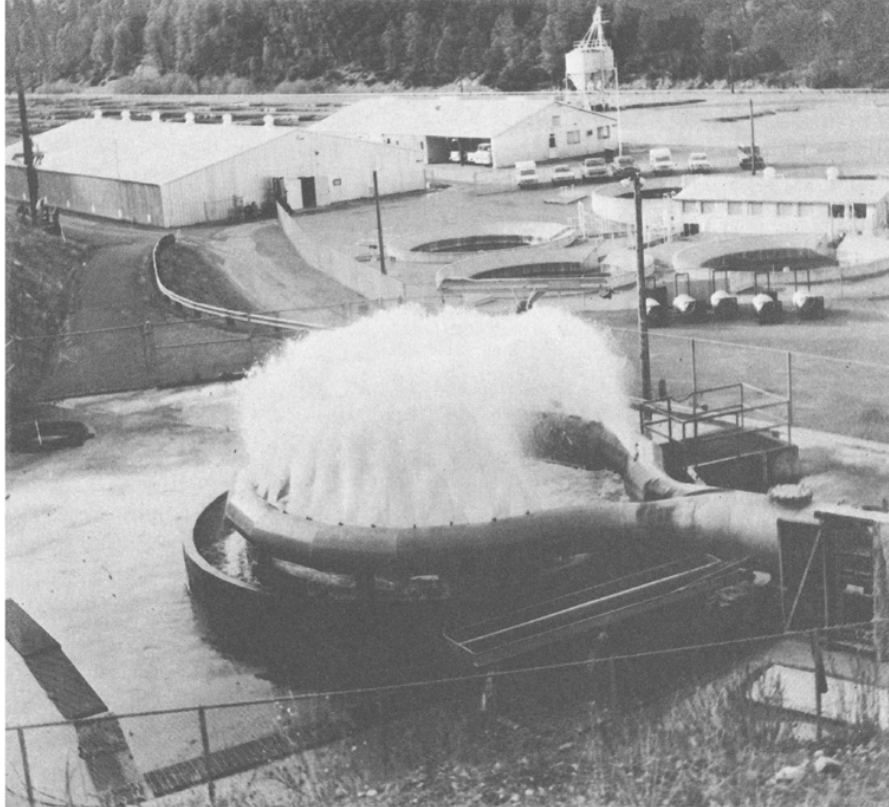
FIGURE 2 —A doughnut type aerator at Trinity River Hatchery, Lewiston, Trinity County, California. The water is sprayed from a circular pipe and falls into a center catch basin to dissipate undesirable gases and add oxygen to the water. Photograph by George Bruley, 1973.
