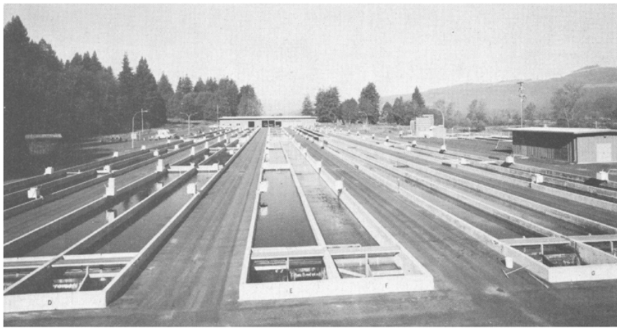
FIGURE 5—Mad River Hatchery, Arcata, Humboldt County, California. Hatchery operates on 30 cfs of water, 90% of which is reconditioned. Only 3 cfs of supplemental water is added to the system. Photograph by George Bruley, 1973.
