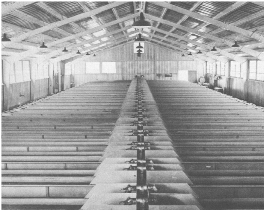
FIGURE 45—Aluminum hatchery troughs. Center water supply permits unobstructed aisle between troughs from one side of building to the other. Photograph by Harold Wolf, 1958.
