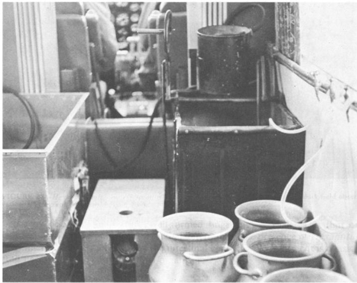
FIGURE 76— A , loading airplane with 5 gallon aluminum cans containing fish to be planted; B , air is supplied to each can in the airplane through manifold and hoses on right side from an electrically driven air compressor in center of picture; hopper from which fish are dropped is at right of picture. Photographs A by Edwin P. Pister and B by George Bruley, 1973.
