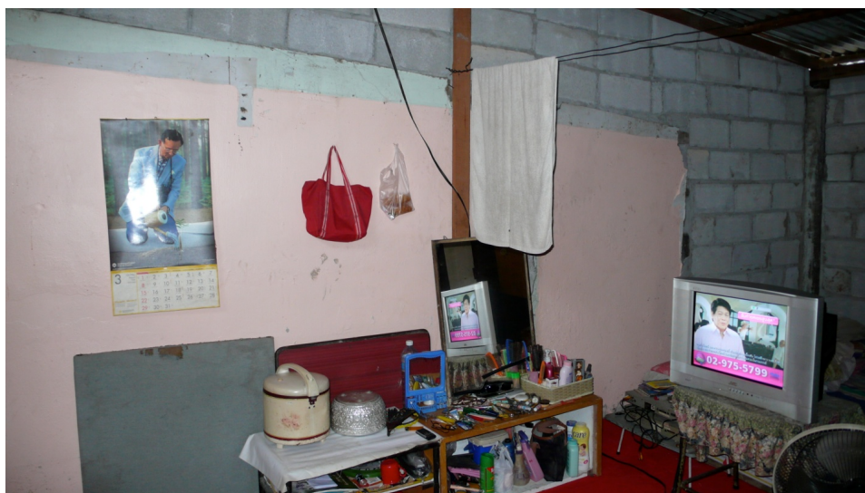
Figure 5.12: Interior of the same house with both old and new walls visible. Source:
