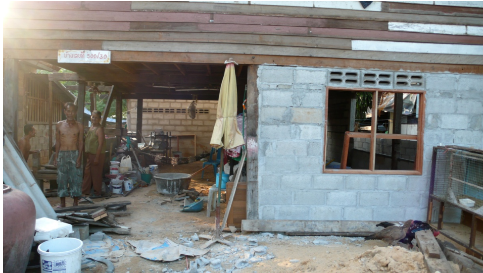
Figure 1.5: Homeowners along the tracks use Baan Mankong funds to enclose their first floor with concrete bricks.
