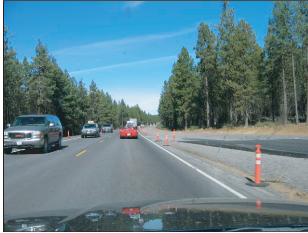
Figure 2. Predicting traffic volume is important when considering terrestrial passage needs within the functional lifespan of a proposed water conveyance structure. Although gravel only few decades ago, this highway has a current ADT at this location of 22,760 and is projected to be 38,700 by 2028 (Oregon DOT). Photo S. Jacobson.
