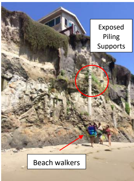
Figure 30. Section 5, Tsq. Isla Vista, Camino Pescadero Beach Access Stairs. Note exposed pillar supports, overhanging mat like vegetation, and people at cliff base for scale (1.75m).
