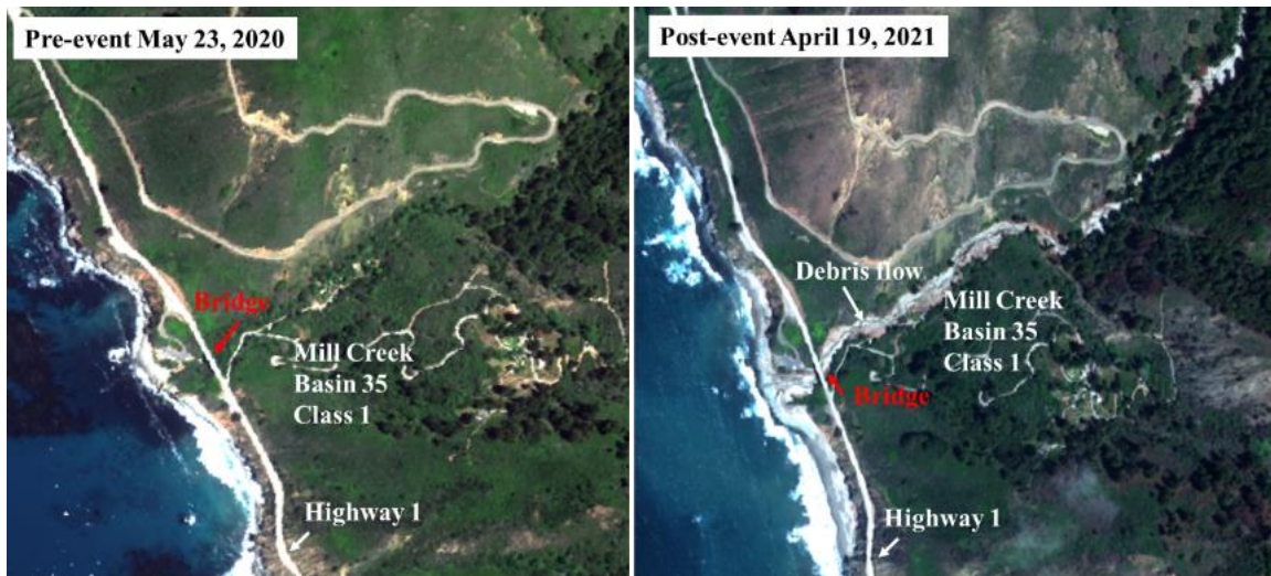
Figure 5.5: WorldView© Imagery (WorldView© 2021, DigitalGlobe, Inc., a Maxar company) at Mill Creek on May 2020 and April 2021 illustrating the occurrence of a major debris flow event that passed below the bridge and thus did not affect the highway performance
