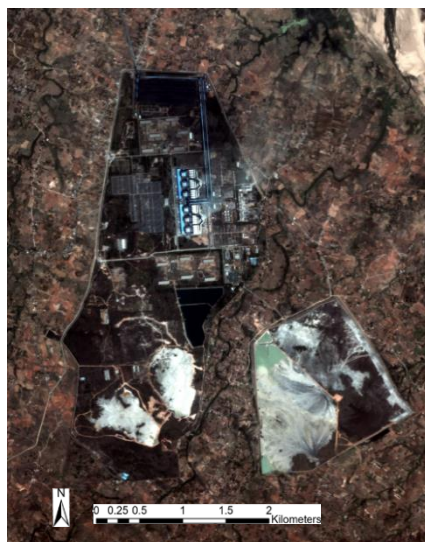
(a) April 09, 2020 (pre-failure)
