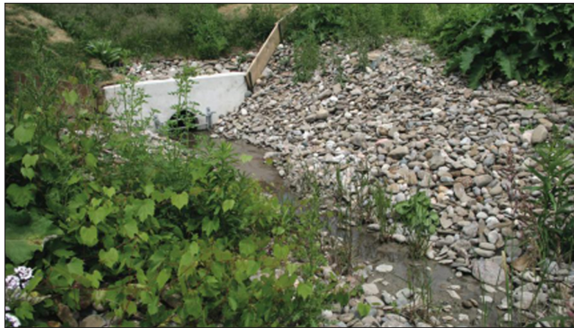
Figure 6. Storm water outfall retrofit to promote infiltration.
