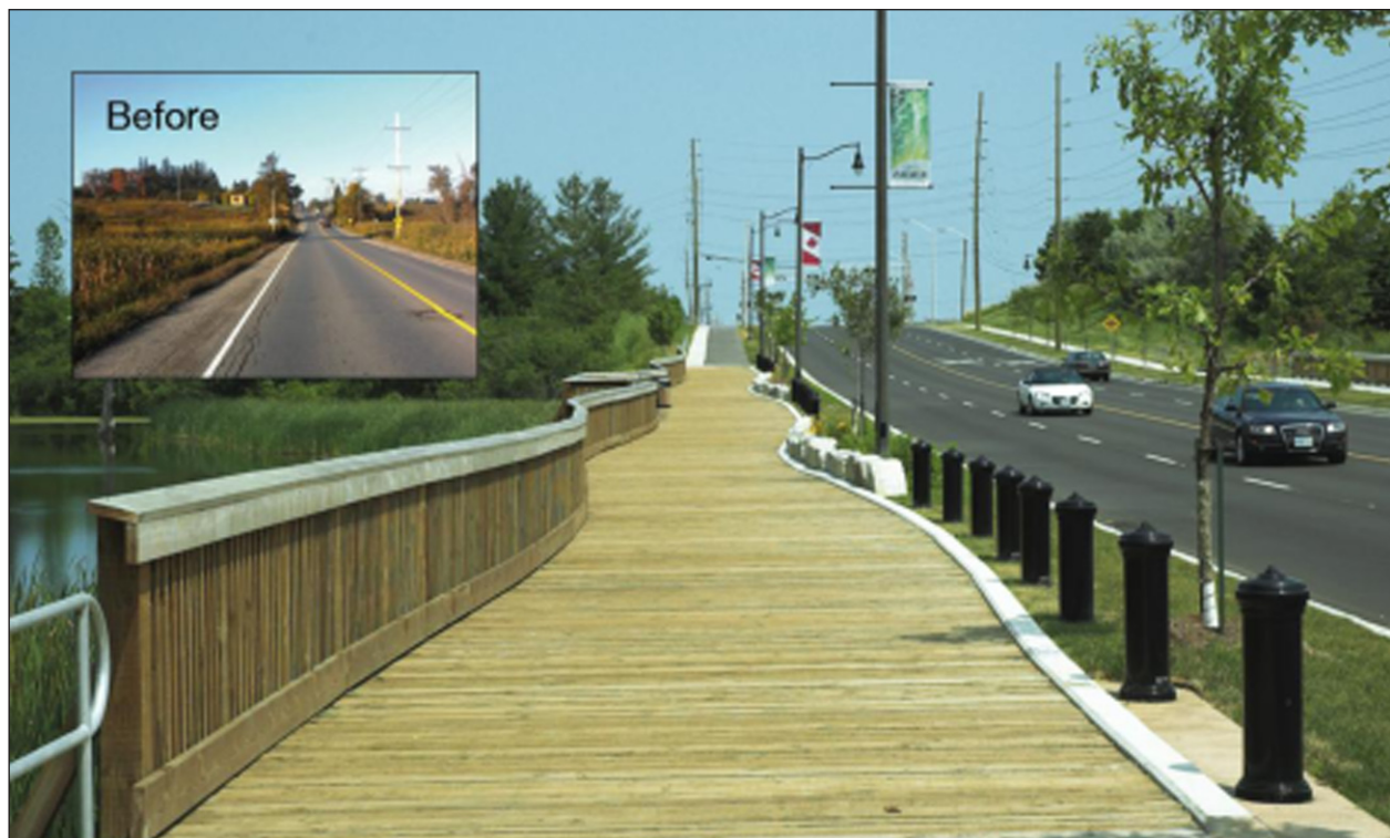
Figure 13. Before and after pictures of the St. John's McKenzie Wetland project.
