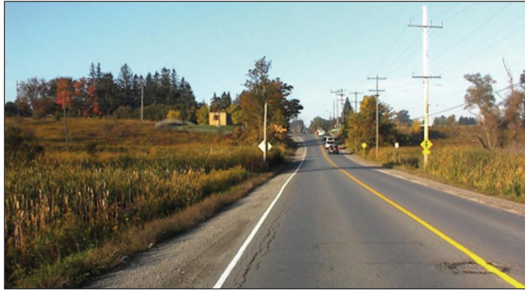
Figure 1. St. John’s Sideroad prior to construction looking west across the McKenzie Wetland.
