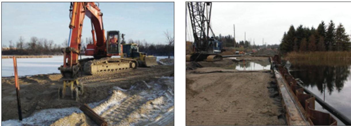
Figure 11. Road platform and the sheet-pile retaining wall under construction.
