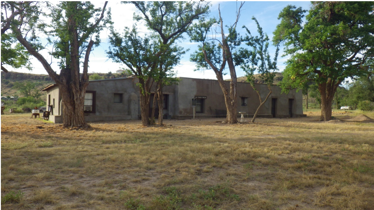
Figure 4.10: Smith-Carlton Casa Vieja in 2014. The main adobe structure is to the right while the main entrance is the enclosed breezeway chapel. The line of trees in front of the house are the remains of a former fence line.
