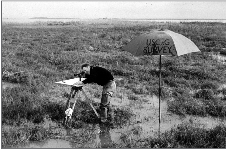
Figure 6 Plane table mapping, Sacramento Delta. (Courtesy of NOAA Central Library.)
