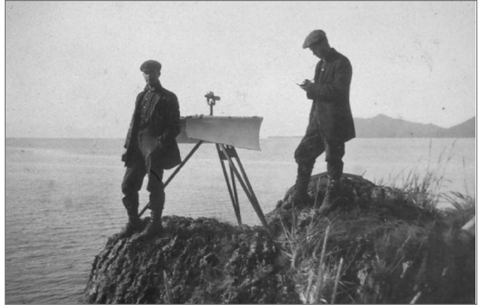
Figure 3 Topographic mapping with a plane table and alidade on the Pacific coast, US Coast and Geodetic Survey. These maps and field notebooks are now at the National Archives and Records Administration II (NARA II) in College Park, Maryland. (Courtesy of NOAA Central Library.)
