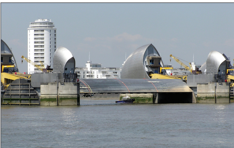
Figure 2. Thames Barrier, with one gate raised for maintenance. The Thames Barrier consists of a series of moveable walls, built in response to a major North Sea flood in 1953. The Barrier protects valuable land in central London. Its walls rotate into place between towers placed at approximately 200-ft intervals across the Thames River near Woolwich, in response to storm surge predictions. Plans are being discussed to replace or enlarge the barrier as sea levels rise (see Reeder and Ranger 2011), which will be extremely costly.
