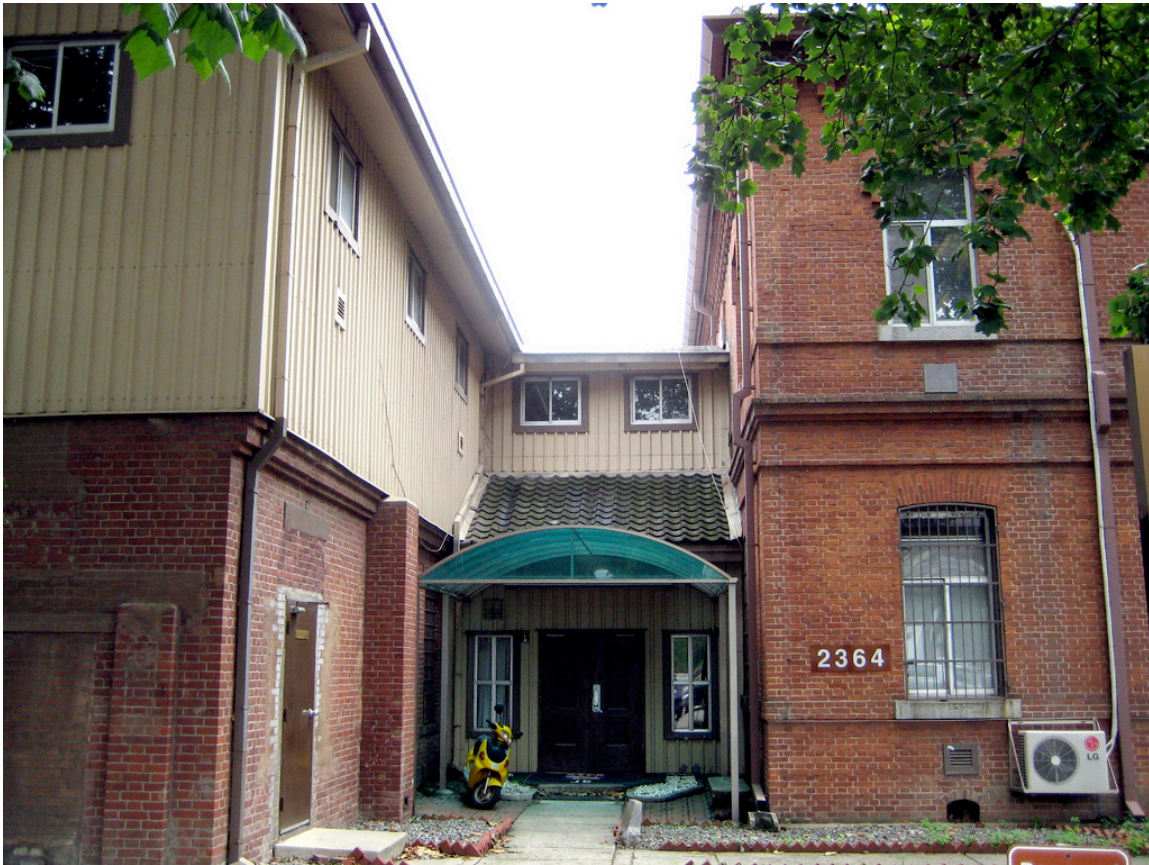
Building 2364: American modification literally built on top of Japanese colonial brick structure, Yongsan
