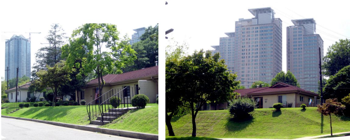
One-story officers' homes replete with lawns juxtaposed to Korean apartment homes bordering Yongsan compound.
