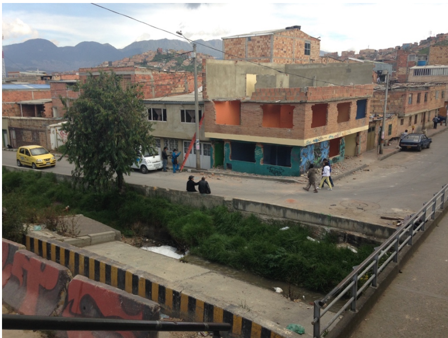
Picture 2. Partially demolished structure in San Francisco next to Quebrada Limas
