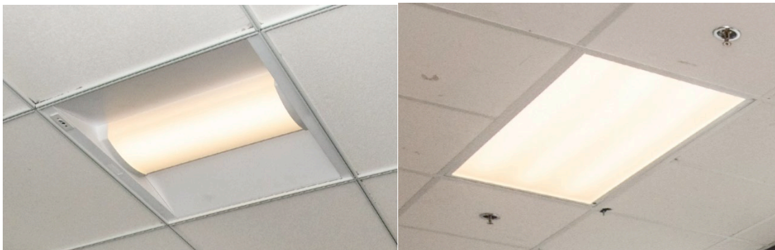
Figure 5. Luminaires used in the tests: LED luminaire used in the ZNE cell (left) and fluorescent troffer used in the reference cell (right).
