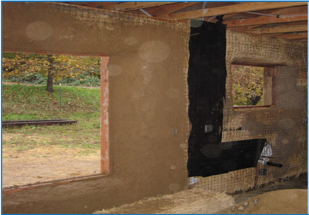
Figure 40: Straw bale Installation around Kitchen Grey Water System in PPN Home
