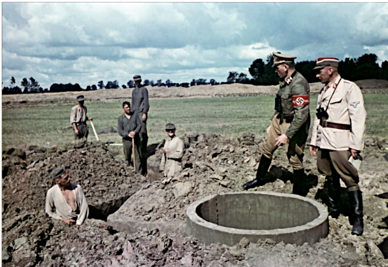
East Prussian volunteers construct Erich Koch's Ostwall, July 1944. 6
