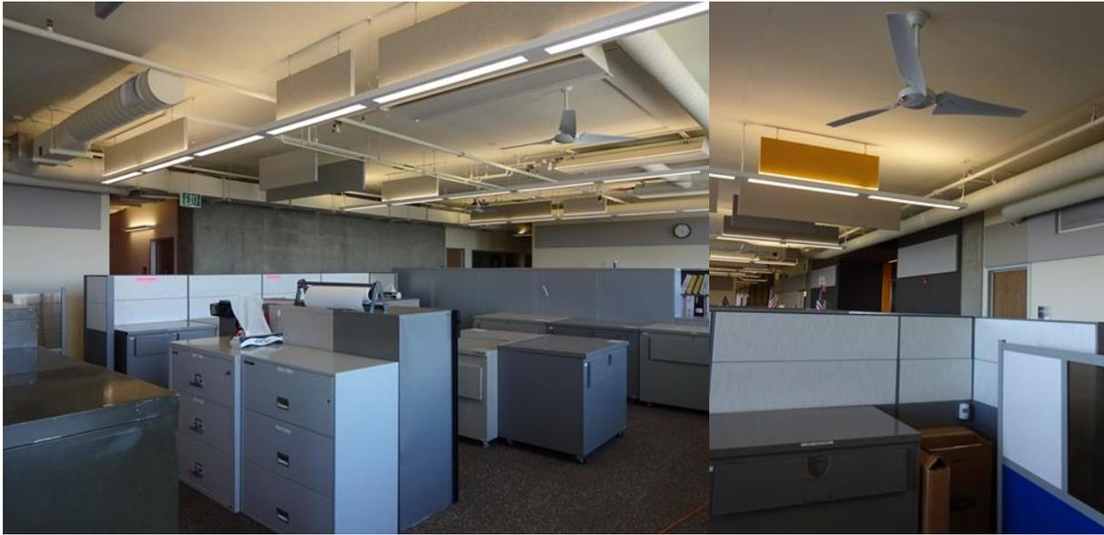
**Left: Open office space with radiant ceiling, ceiling fans and overhead mixing diffusers for ventilation only. Right: Ceiling fan over open office cubicle.**
