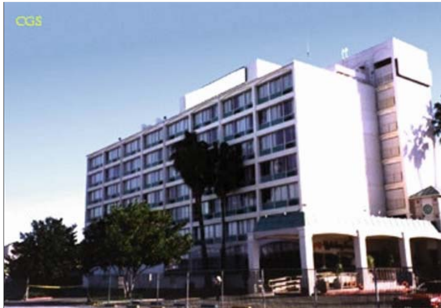
Figure 1.3: Holiday Inn Van Nuys, California seen from distance after 1994 Northridge earthquake.
