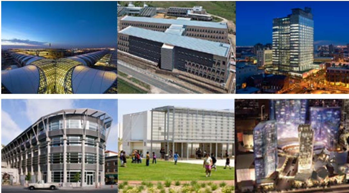
Figure 1-1: Examples of buildings with radiant systems installed 1
