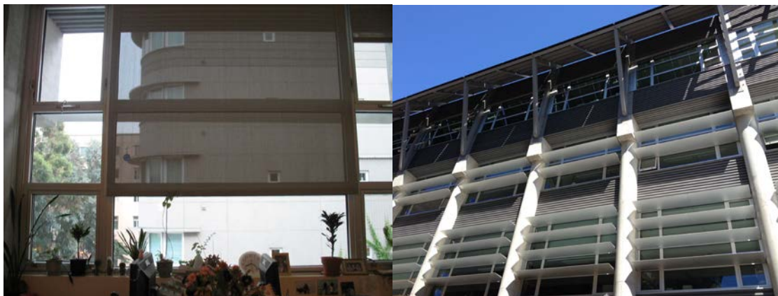
Figure B-1: DBC interior roller shade (left) and exterior fixed shades (right) on south façade
