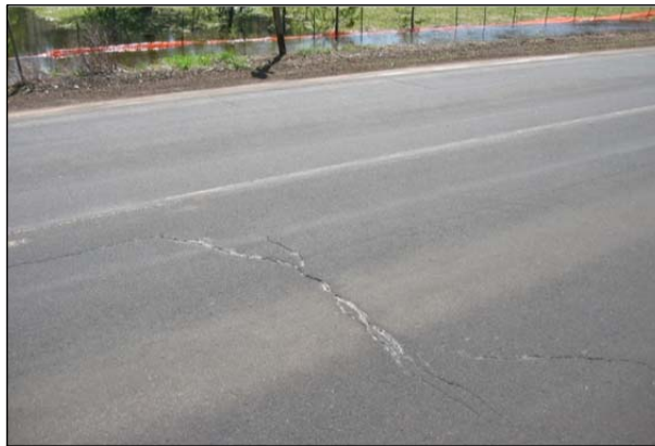
Figure 2.1: Transverse crack.
