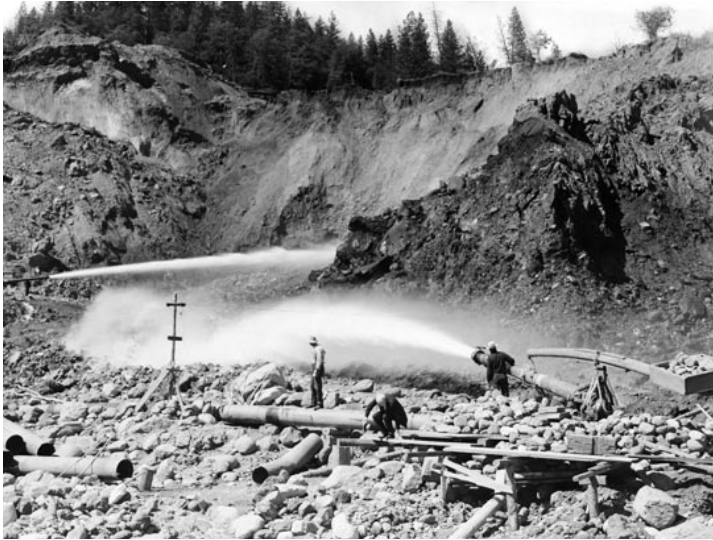
Figure 2. Hydraulic mining, 1860–1870, Trinity County. Streams were diverted through flumes, ditches, and pipes to monitors (nozzles) to wash gold-bearing gravels into sluice boxes for separation of the gold. Source: Eastman's Originals Collection Group 117, Special Collections, University of California Library, Davis, reprinted with permission.
