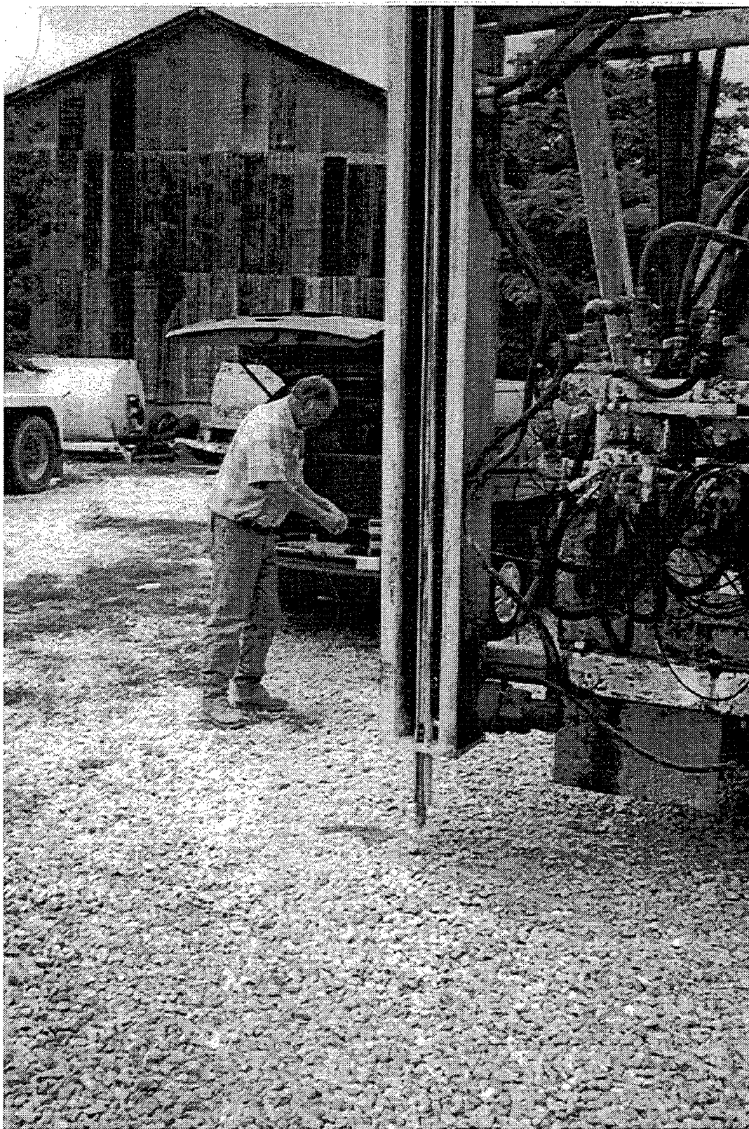
Figure 3. Lance injection truck with instrumented injection tip installed. Masthead is locked in the vertical position.
