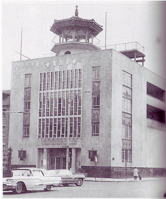
Figure 3: The Chinese Merchants Assoc. building, remodeled after its back end was demolished for the Central Artery in 1952.
