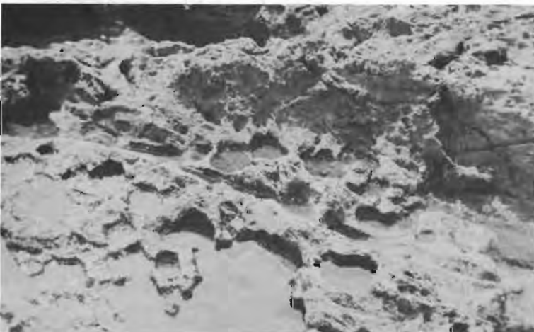
Figure 18. Solution basins in Miocene basalt near Resort Point, Palos Verdes Hills. Basins are believed to form by biochemical methods like those in sandstone and limestone. Photographed May 1956.
