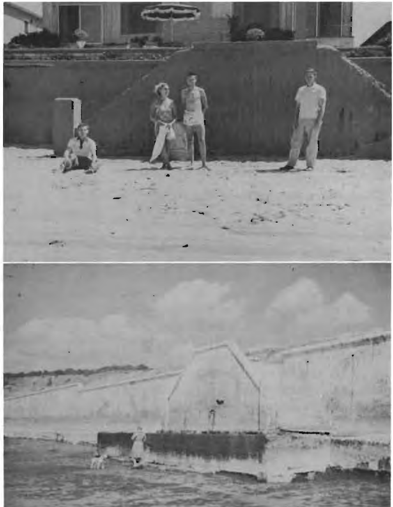
Figure 29. Change of beach north of La Jolla. In the top photograph taken in August 1955 a broad sand berm has been built and the sand is piled high against the sea wall; in the bottom photograph taken in February 1942 the sand had been completely stripped from the beach and the waves had exposed the underlying terrace material. Courtesy F. P. Shepard.
