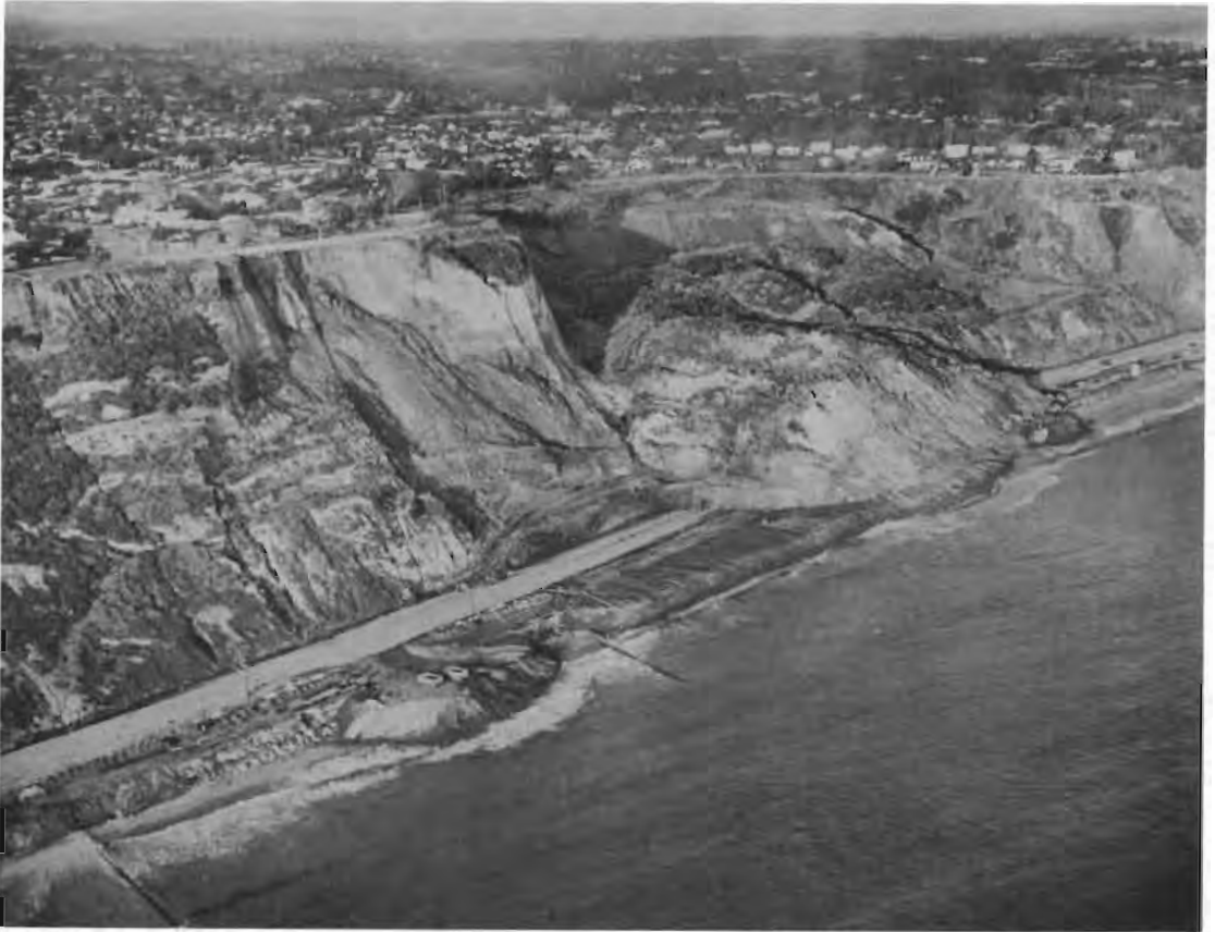
Figure 239. Landslide of April 1958 at Pacific Palisades west of Santa Monica which cut off coastal traffic for several weeks. It occurred just as a previous slide (to its left) had been nearly cleared up by dumping along the shore. Movement was so unexpected that it caused one death and the destruction of several pieces of earth-moving equipment. Compare with Figure 20, Section 7. Photograph by Pacific News Pictures.
