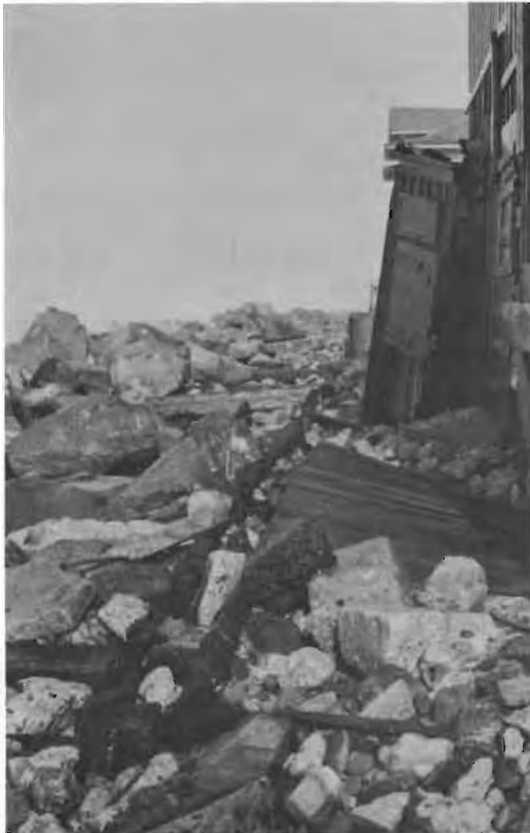
Figure 10. Wave damage to house at Redondo Beach. Photographed January 17, 1953, after a small storm.
