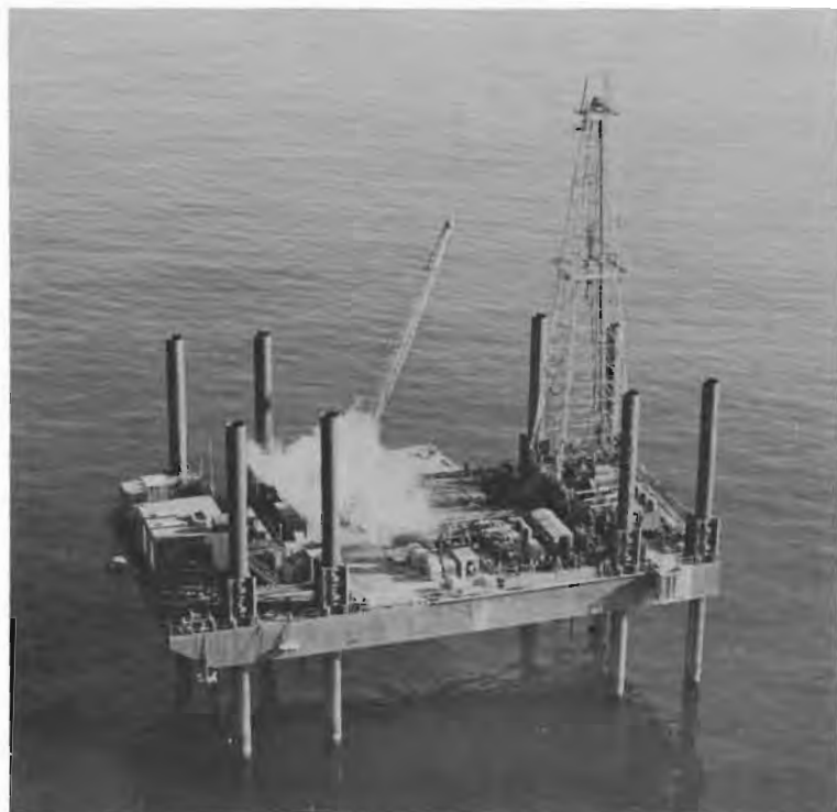
Figure 246. Texas tower type of offshore drilling platform being used off Huntington Beach in 1957. Courtesy of Howard C. Pyle, Monterey Oil Company.
