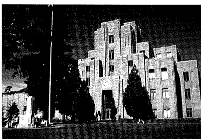
PWA-era courthouse in Boulder, CO. Courtesy Todd W. Bressi.
