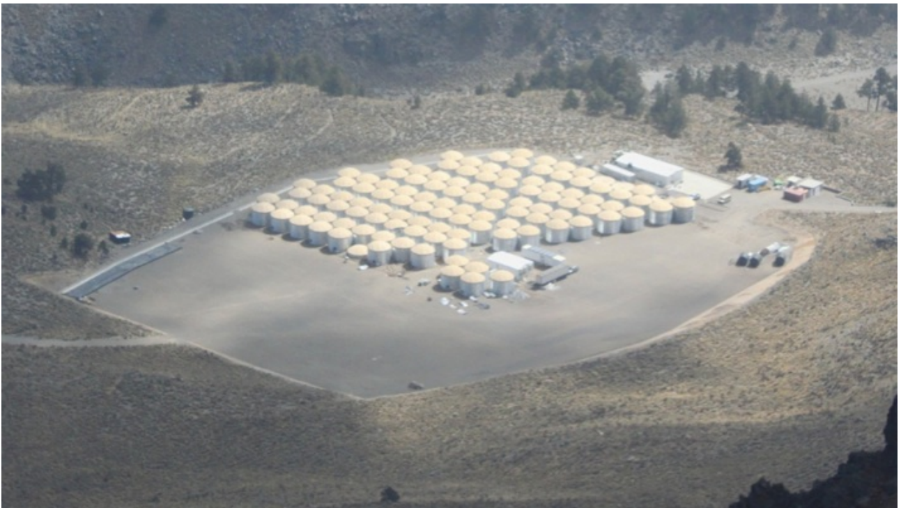
Figure 4: View of HAWC with over 100 tanks (May 2013).
