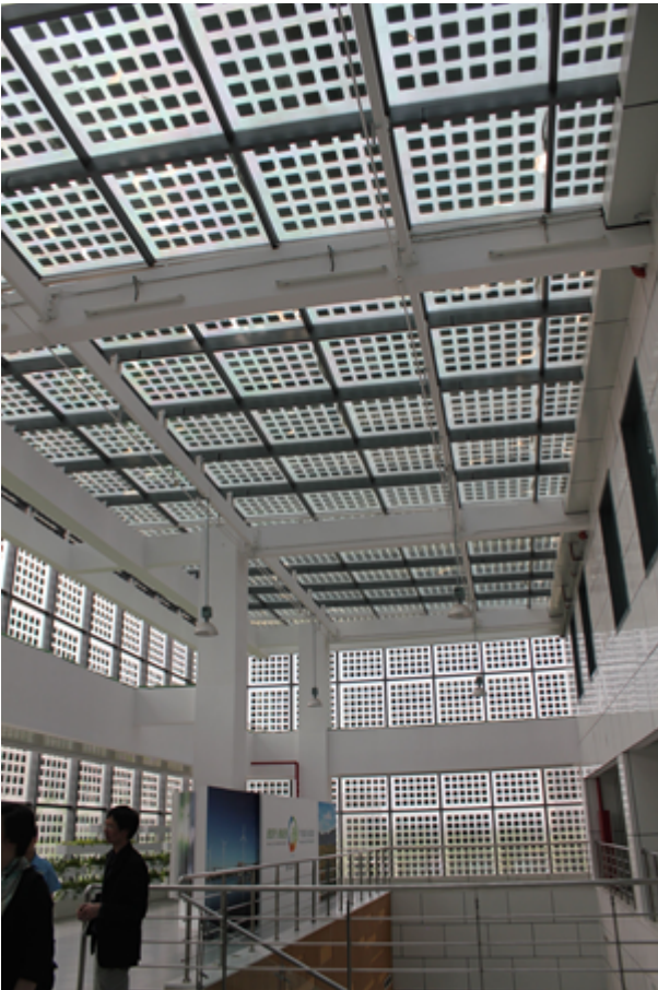
Figure 3.4. Translucent PV at TEC
