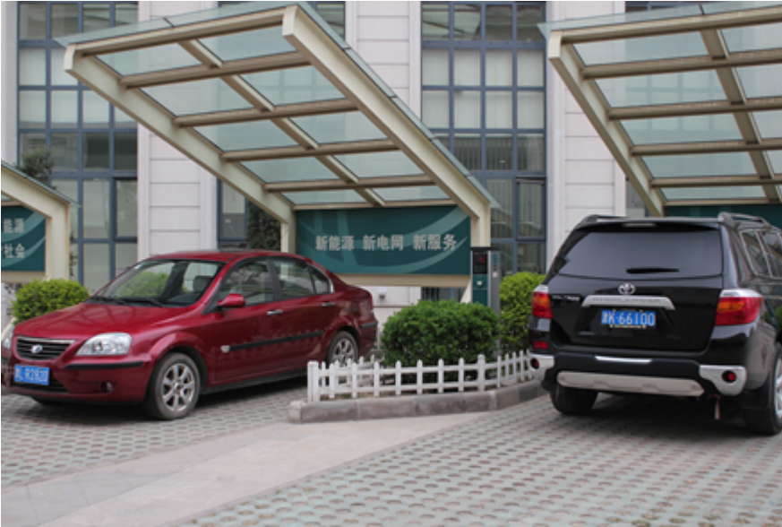
Figure 3.3. EV charging stations at TEC microgrid
