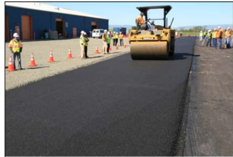
Test track compaction
