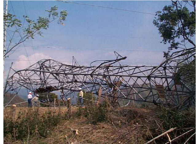
Fig. 1 – Transmission tower destroyed by attack. Photo courtesy of Interconexión Eléctrica S.A. E.S.P. (ISA).
