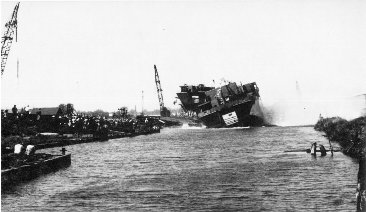
Launching of the Melville , sideways, at Defoe Shipbuilding Company, Bay City, Michigan, on 10 July 1968. Photo by James Pollock.
