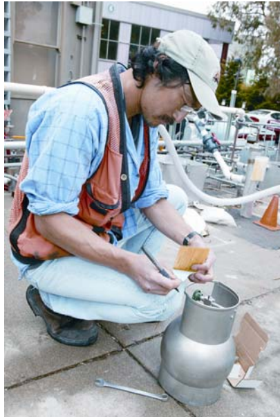
Collection of a gas sample from a soil vapor extraction system near Building 7
