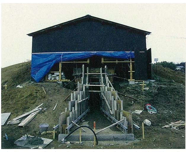
Figure 37. Construction of a modern entrance into the Fujinoki tumulus. (Ikarugachō Kyōiku Iinkai, *Shiseki Fujinoki Kofun hozon seibi jigyō hōkokusho*, 117)
