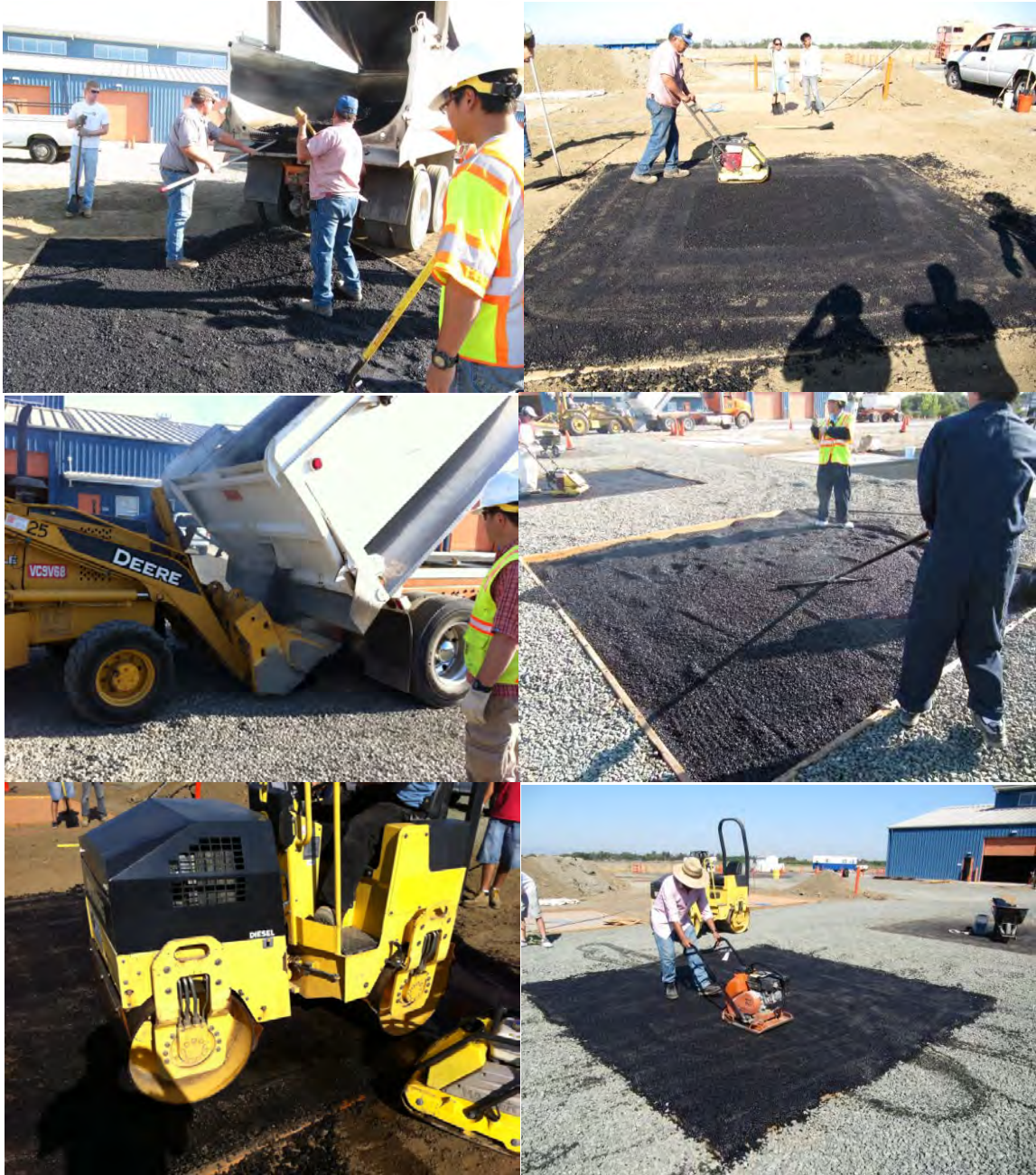
(e) Construction of surface layer (asphalt pavement).
