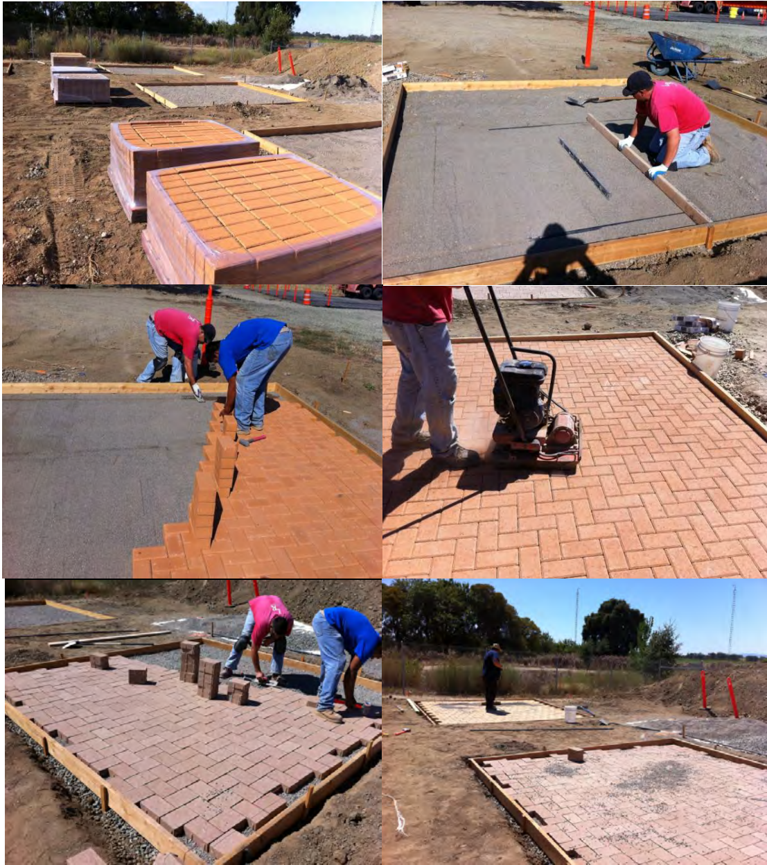
(c) Construction of surface layers (paver pavements).
