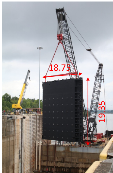
Figure 5.8. Picture of a lifted miter gate at Greenup
