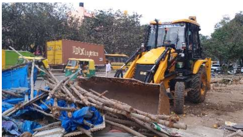
Figure 22: JCB excavators demolishing the marketplace
