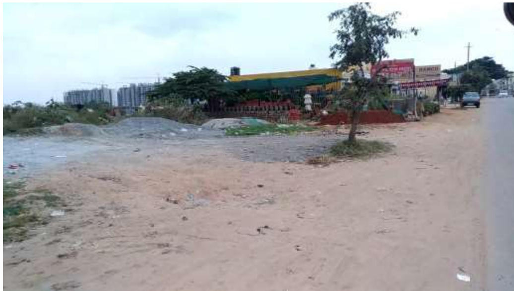
Figure 2: Urban transformation along Central road. Empty erstwhile farm lands, condominiums under-construction and small local business dot the length of the road
