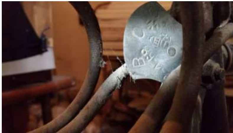
Figure 51: BCC stands for the Bangalore City Council, which was the then municipality. The last stamped date on the plate is “1-4-68”
