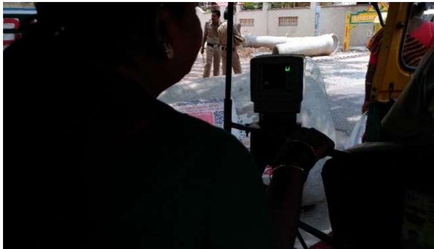
Figure 28: Road repair work holding up the traffic and Vijayalakshmi's friend alights here
