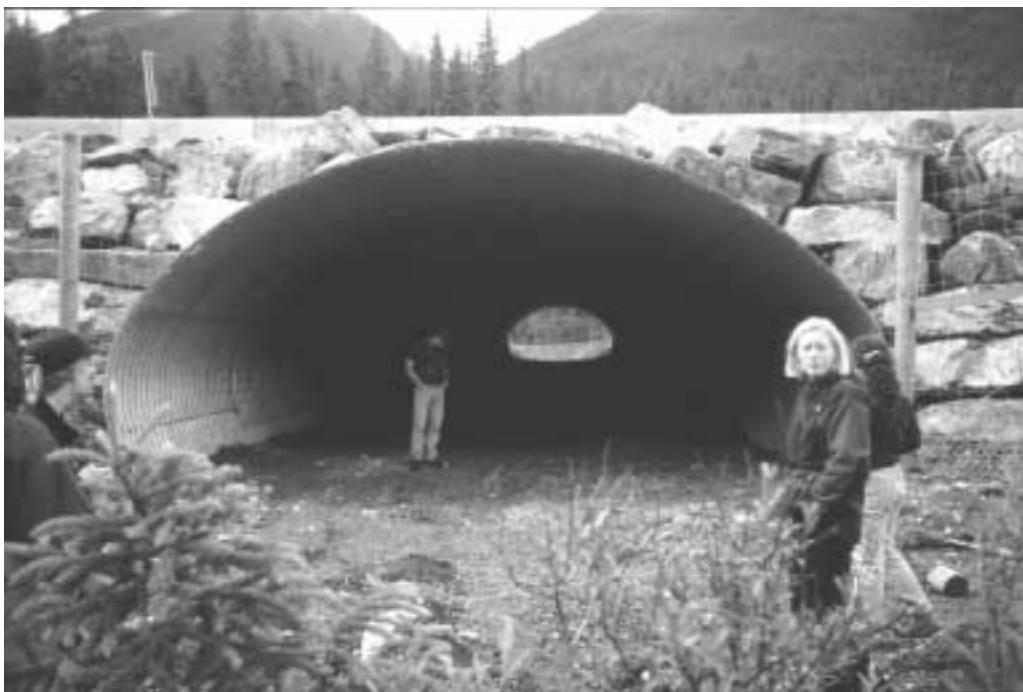
Fig. 2. Steel Arch on Trans-Canada Hwy in Banff National Park. Structure is large, but still has more "tunnel effect" than span in Figure 1. Some mobile species like deer and elk readily accept these structures. Other may be intimidated by the "tunnel effect."
