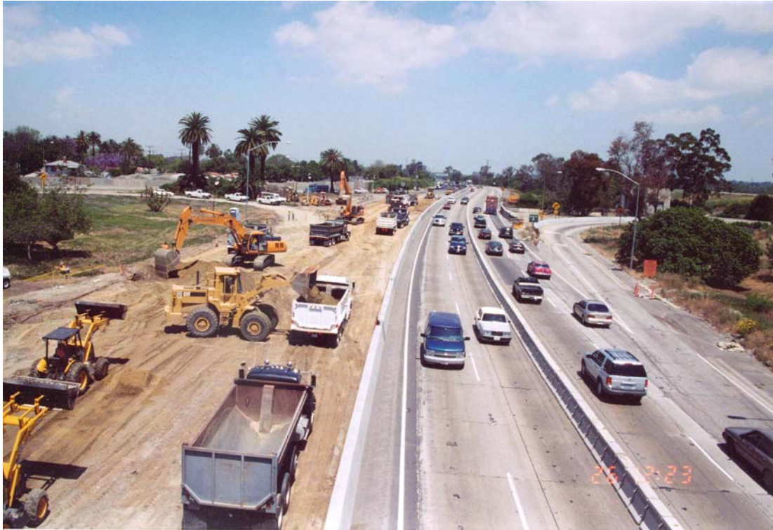
Figure 3. I-710 rehabilitation and traffic control during the weekend closure.
