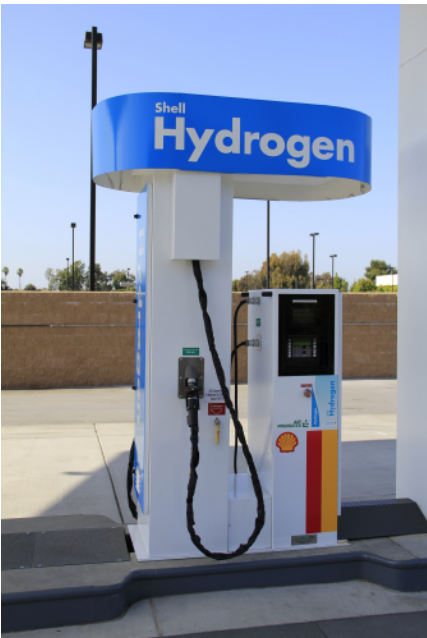
FIGURE 18.4.1 The first California hydrogen fueling station fed directly from an active industrial hydrogen pipeline. Photograph from US Department of Energy.
