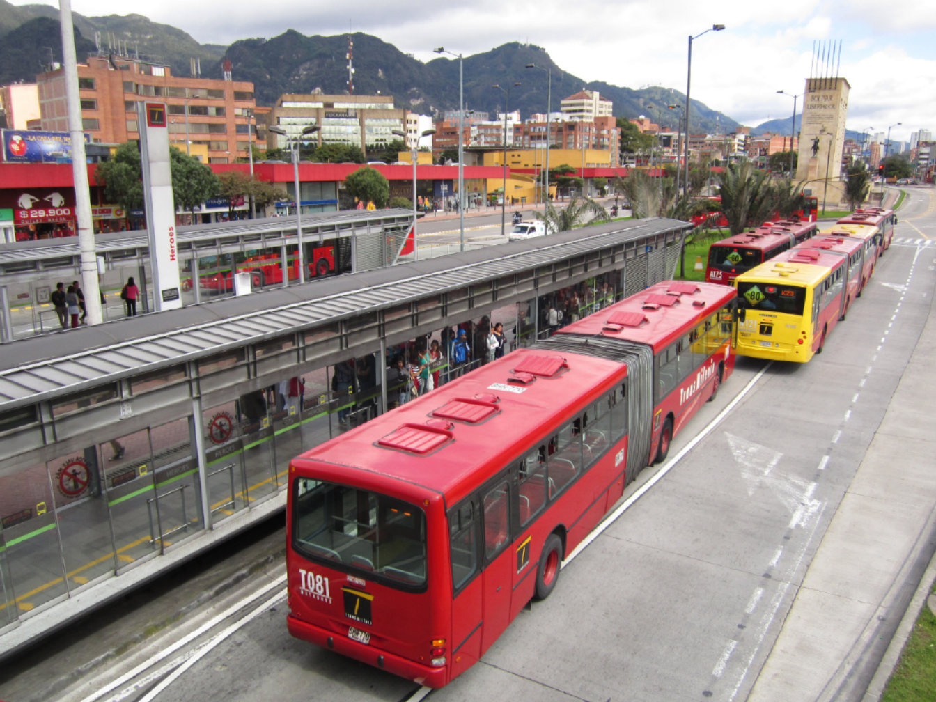
FIGURE 6.3.2 Bogotá's Transmilenio bus rapid transit (BRT) system in the early 2000s became a model for BRTs. Photograph by Felipe Restrepo Acosta on Wikimedia Commons.
