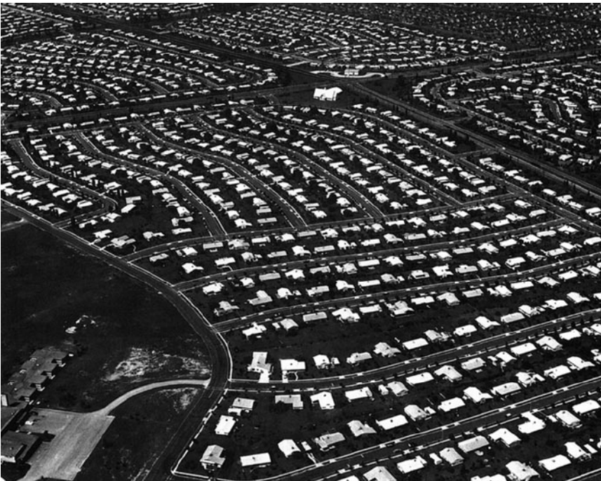
FIGURE 2.2.4 Levittown, Pennsylvania, was the first master-planned development in the United States, built in the 1950s. Its 17,000 identical houses inaugurated a new symbol of American happiness—the single-family home in the suburbs—that also required freeway infrastructure and an oil-hungry automobile industry. Reproduced from Wikimedia Commons.
