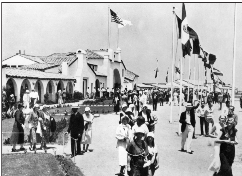
Fig. 7-5: View of Olympic Village Administration Building, 1932 LAPL Security First National Bank Collection (00098667)
