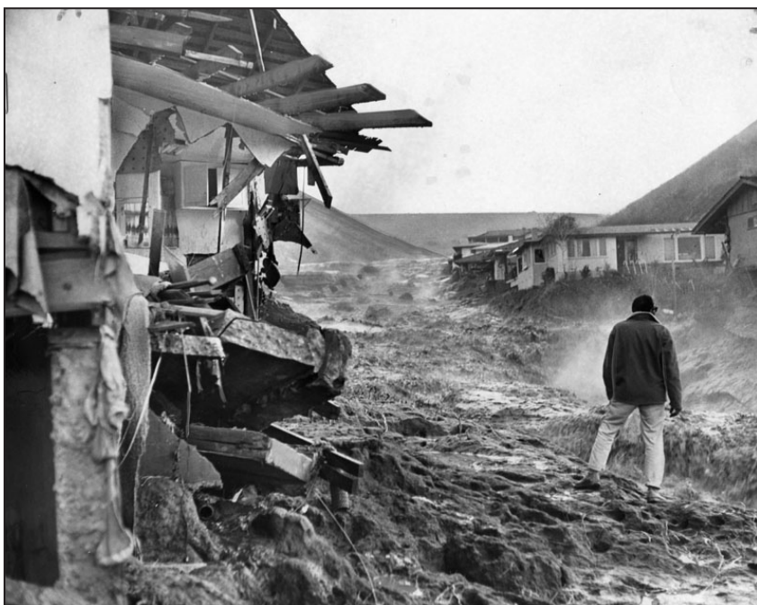
Fig. 7-15: View of the Baldwin Reservoir Collapse, 1963 LAPL Herald-Examiner Collection (00060008)
