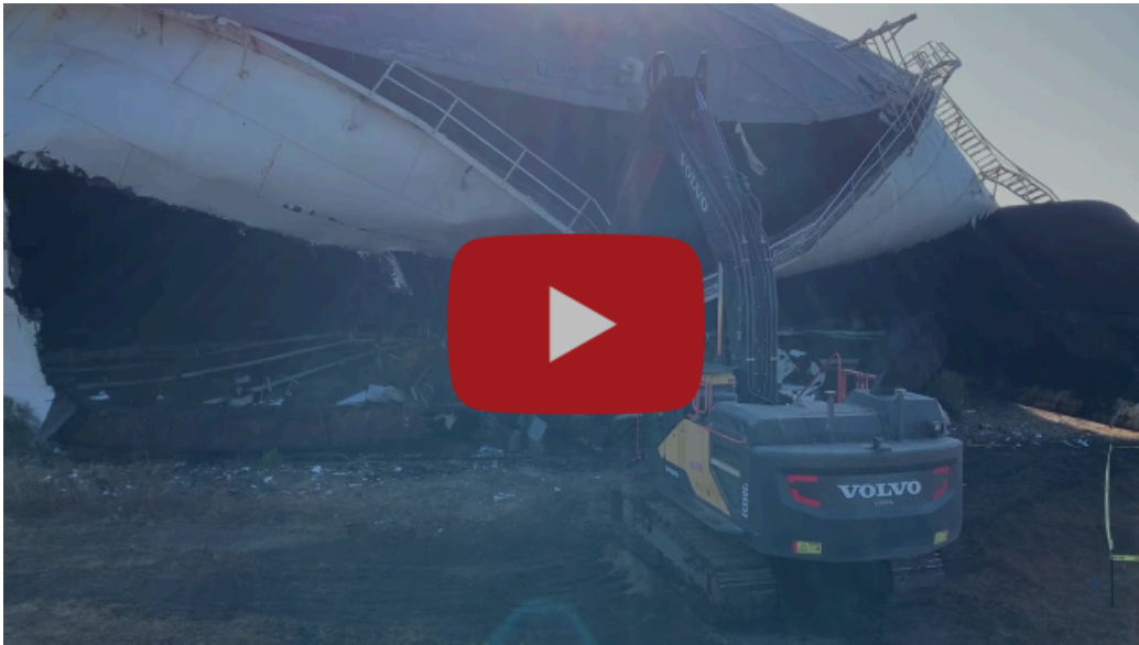
EMT Tank Demolition - 9/11/2024. Video by John Fitzgerald.
