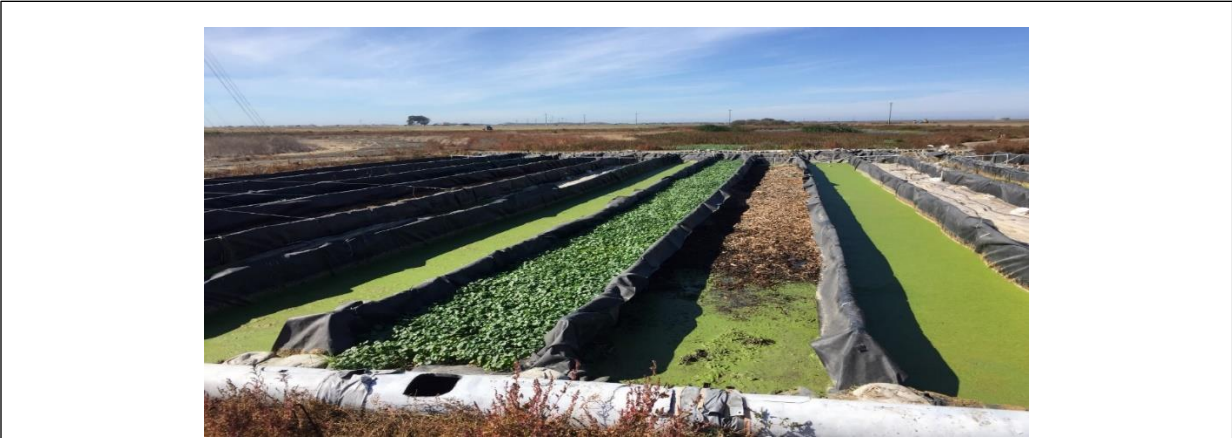
Figure A8. Photograph of PG&E Multichannel Bioreactor, Castroville, CA. There are three woodchip channels at this site, with dimensions 22.6m x 1.68m x 0.762m (LxWxH).
