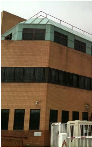
West London County Court, England Micro-shade attached to windows (shd2) (picture: Courtesy of smartlouvre)
