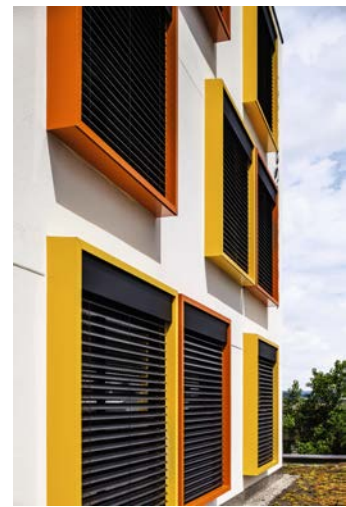
Center for elderly people, Switzerland Curved blinds in roller shade (shd 7) (picture: Courtesy of Warema)
