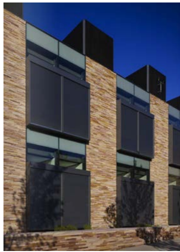
Hilton Foundation, Agoura Hills, USA Stainless steel roller shade (shd 6) (picture: Courtesy of ZGF Architects, LLP; Photograph Nick Merrick © Hedrich Blessing)
