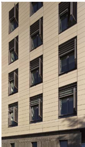
Li Ka Shing, UC Berkeley campus, USA Aluminum louvers above operable windows and in shutters (similar to shd 8) (picture: Courtesy of ZGF Architects, LLP; © Robert Canfield)
