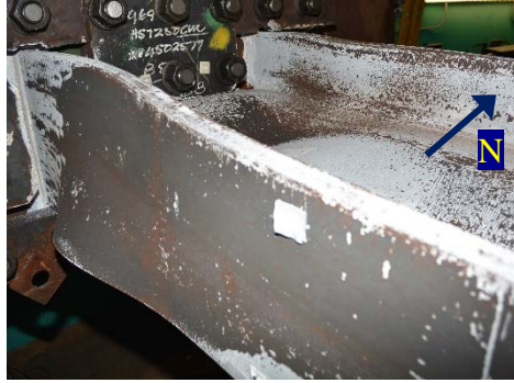
(a) Southwest Flange
