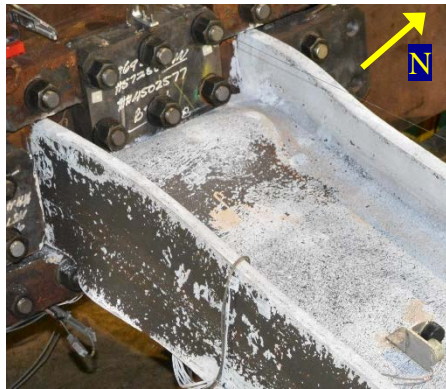
(a) Southwest Flange
