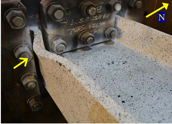
(a) Southwest Flange
