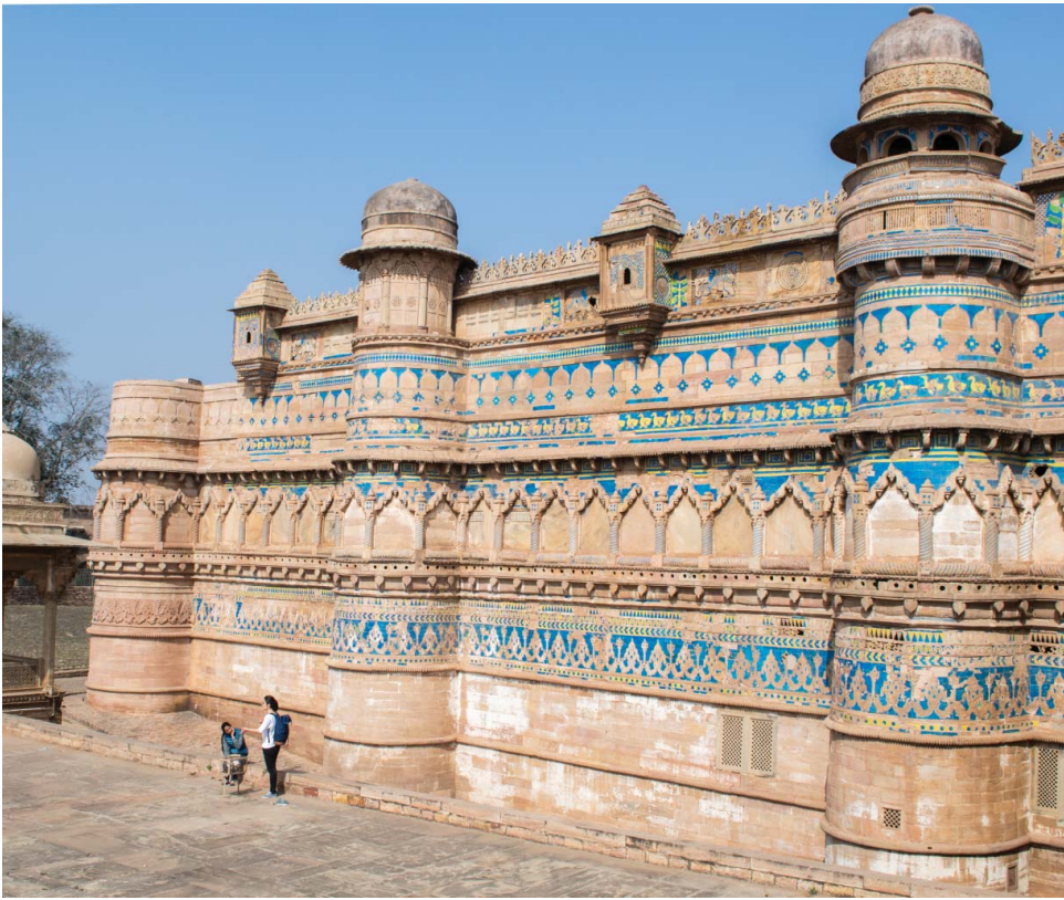
Figure 6. Façade, Man Mandir, Gwalior, c. 1500. Source: Author's photograph, 2014.
