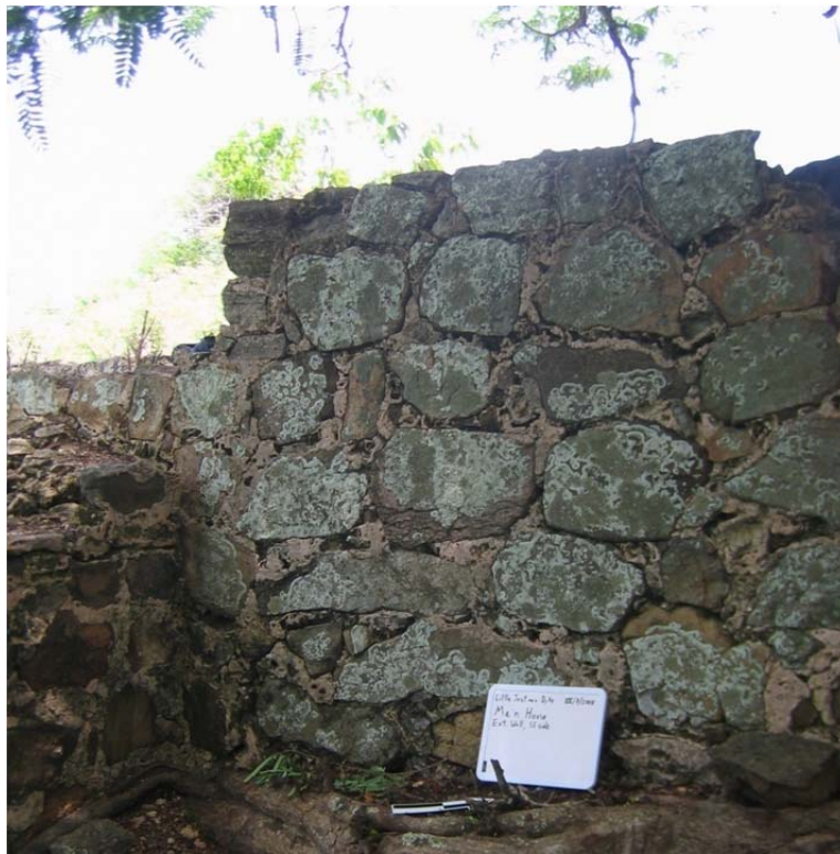
Figure 6.6: Southeast wall of planter house
