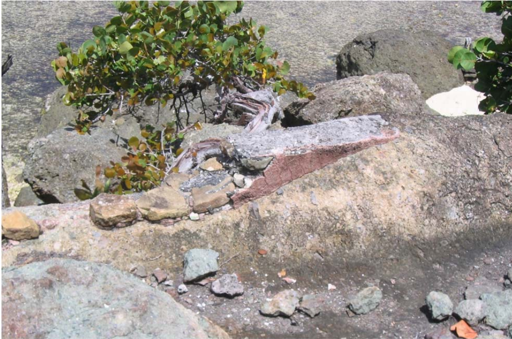
Figure 6.16a: Wall on modified boulder
