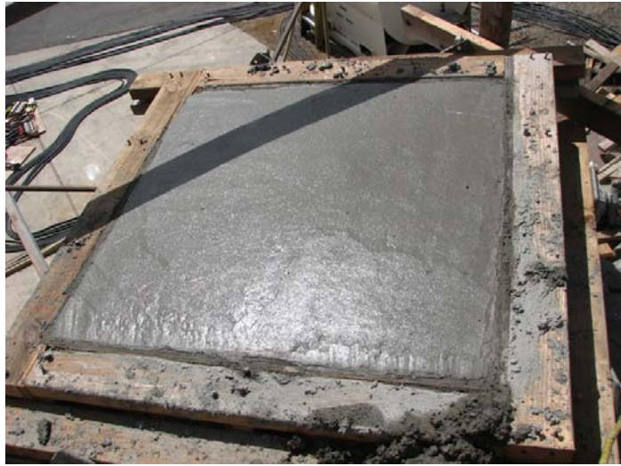
(c) Finished top block surface
