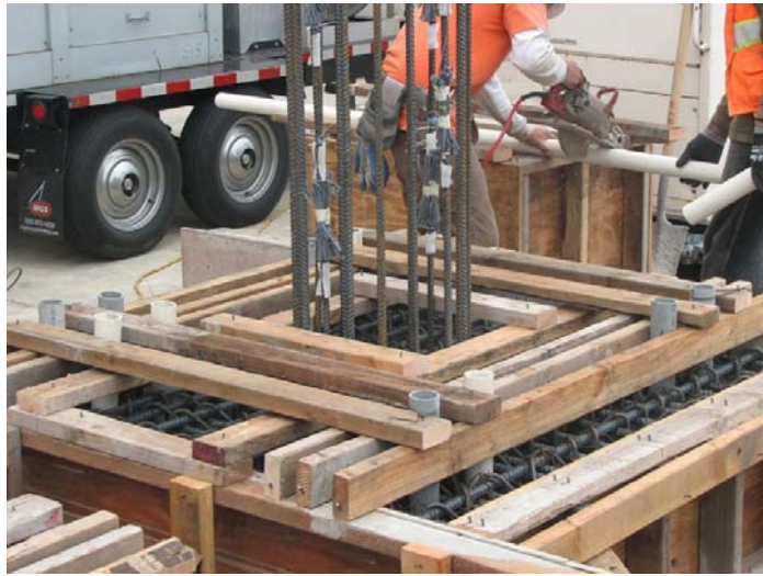
(a) Finishing formwork
