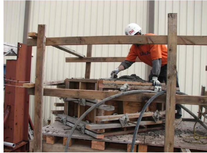
(b) Leveling top block surface
