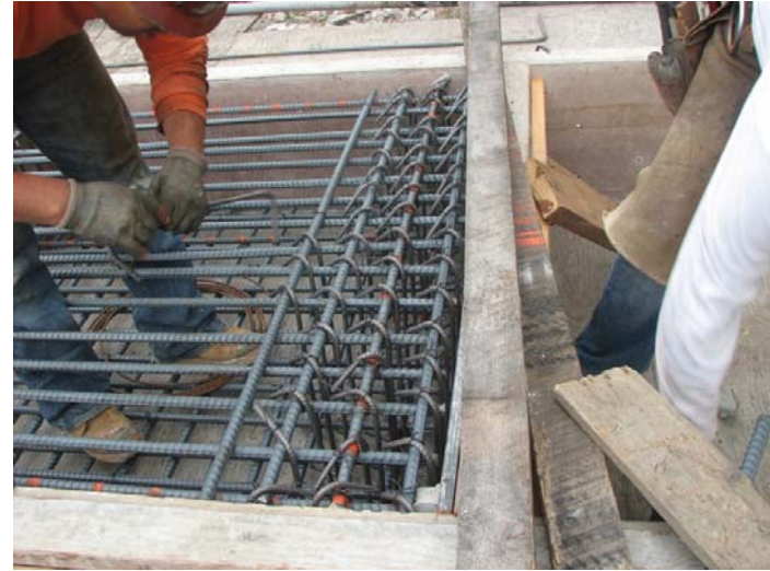
(b) Top and transverse reinforcement
