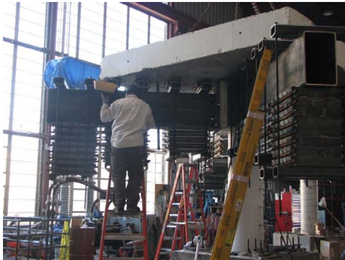
(c) Grouting between the beam and the concrete block
