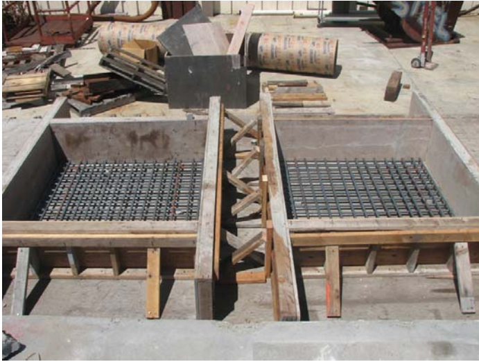
(a) Bottom reinforcement
