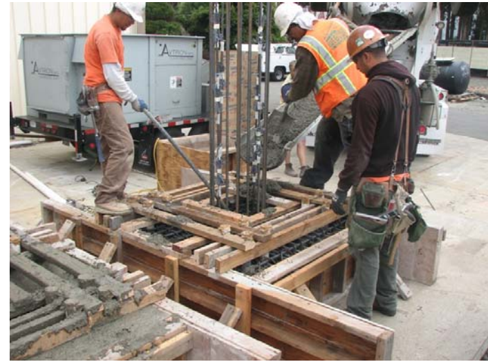
(b) Placing concrete mix
