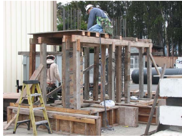
(b) Formwork for top block
