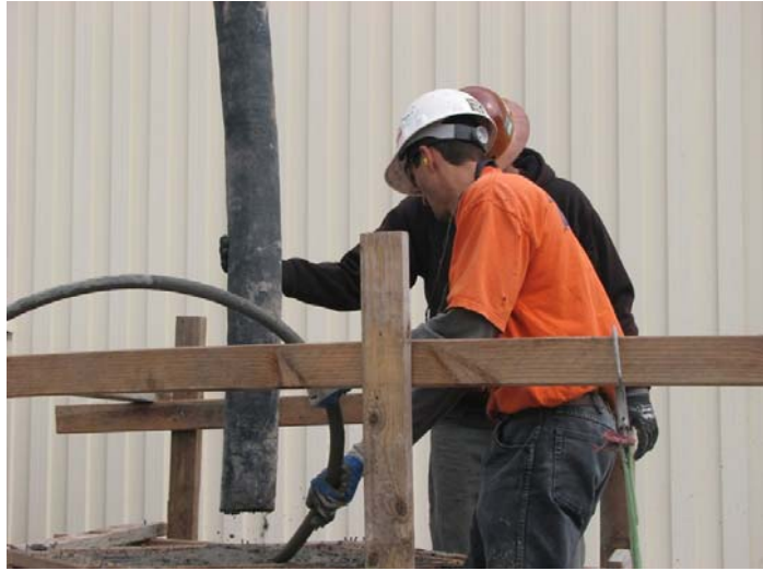
(a) Placing concrete mix
