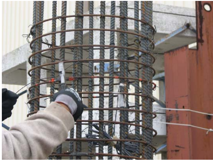
(a) Strain gages on column reinforcement
