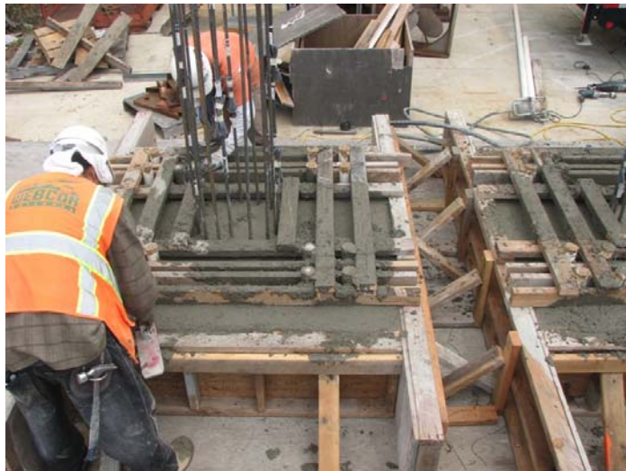
(c) Leveling footing surface
