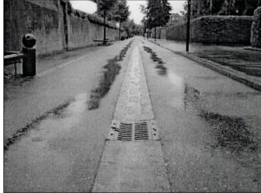
Figure 9. An urban example demonstrating that storm water must not necessarily be collected at the edge of the roadway. For roads leading through more natural surroundings, such a design could serve as a measure to reduce animal mortality in drainage chutes.
