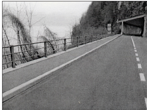
Figure 1. This curbstone is known to guide Amphibians directly into the tunnel.
