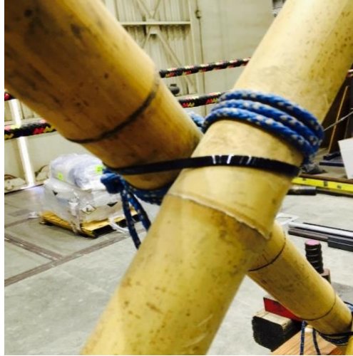
Figure (4.16): Cable Ties Looped Around the Joint
