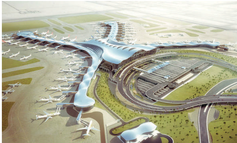
Figure 6.22 Abu Dhabi Midfield terminal expansion
