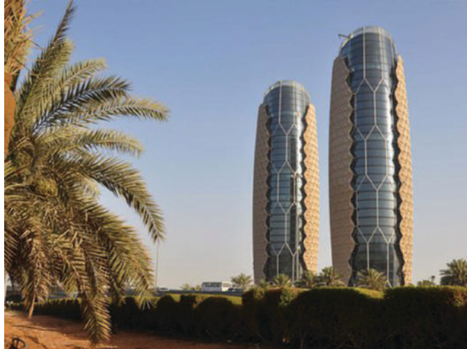
Figure 6.61 Al Bahar Towers
