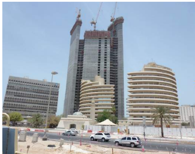
Figure 6.49 Old ADNOC buildings with new HQ tower in the background
