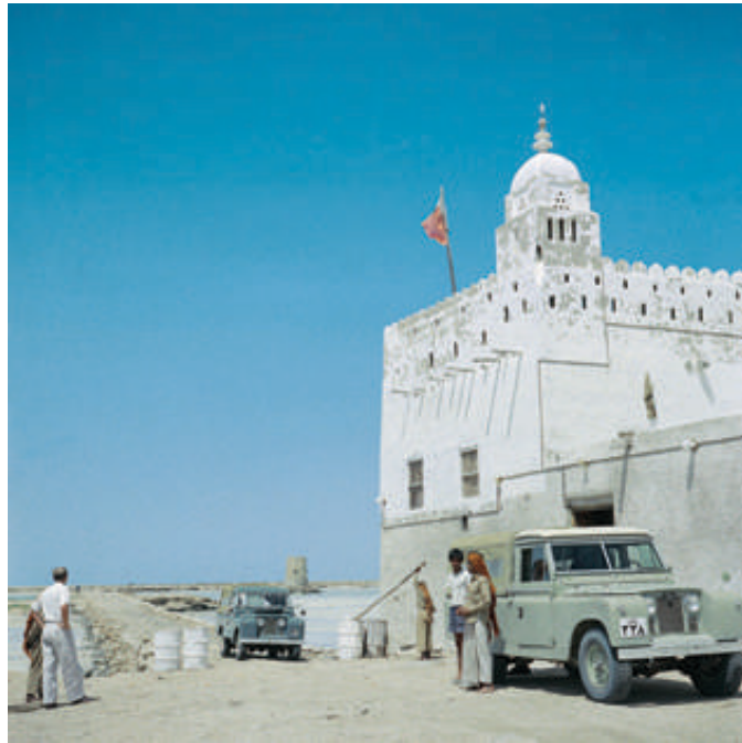
Figure 4.22 Stone causeway, customs post and watchtower.
