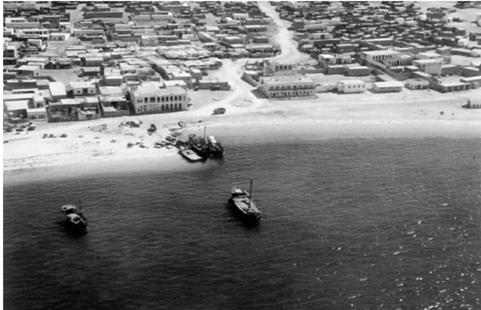
Figure 5.30 Abu Dhabi buildings 1968
