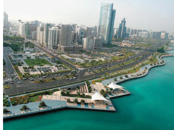
Figure 6.41 Corniche redevelopment c.2008
