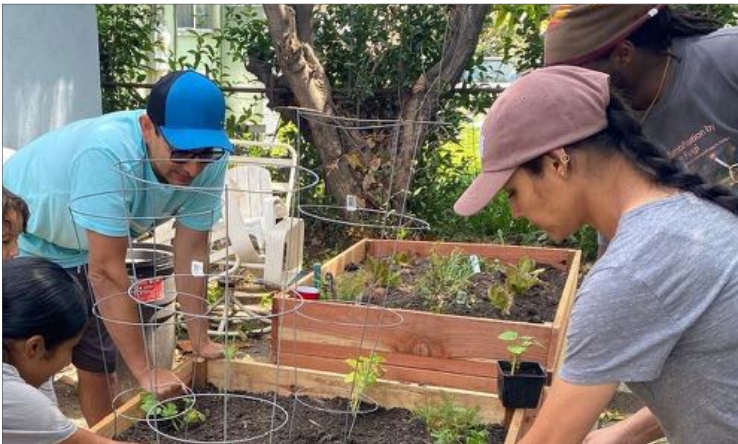
Installation of an urban minifarm at a Watts resident’s home. Photo credit: MudTown Farms Instagram
