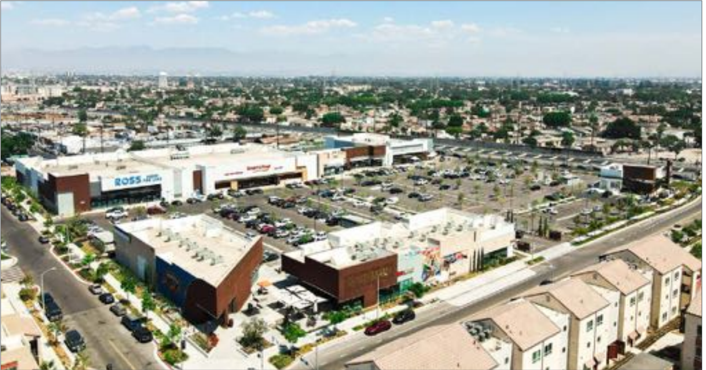
Jordan Downs Phase 1B Retail Center, known as Freedom Plaza. Photo credit: Freedom Plaza Watts.
