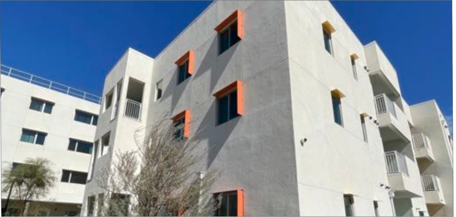
Apartment building of Jordan Downs Redevelopment S2, Sky at Jordan Downs. Photo credit: The Michaels Organization
