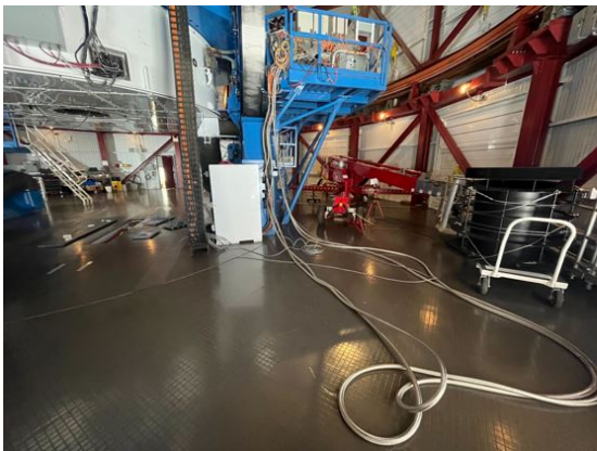
Figure 2.13 Compressor hoses being installed at Clay. (Left) Hoses being routed from the pier to NASE, the blue platform at the top center. (Right) Into the cable wrap after installation.
