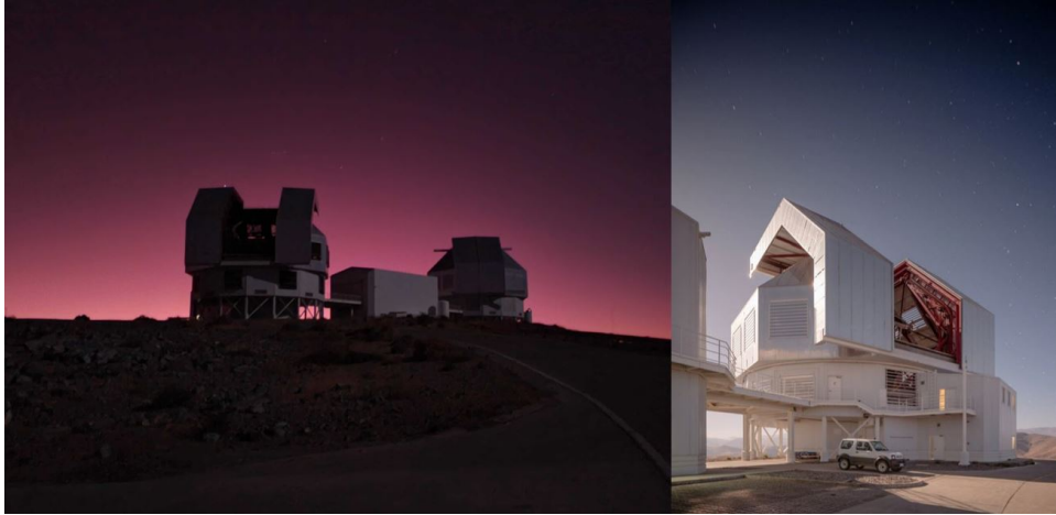
Figure 2.1 (Left) The Magellan Telescopes at dusk from the southeast. The Baade Telescope can be seen in the process of opening for the night, and to the right the Clay Telescope is rotating into position before opening. Between the two is the Auxiliary Building where the mirrors are polished and instrument maintenance is performed. (Right) Courtesy of Overbye (2023). A closer view of Baade Telescope at night.
